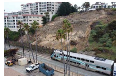
San Clemente Track Protection Project – After
