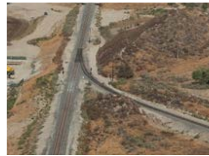
Vista Canyon Station – Before
