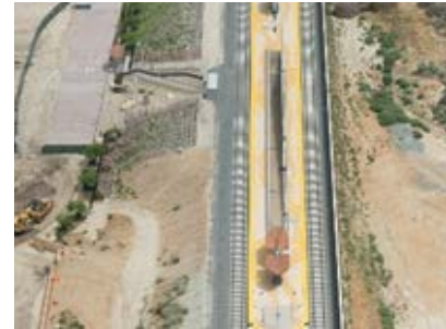
Vista Canyon Station – After
