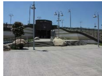
Vista Canyon Station – After
