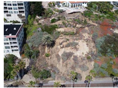
San Clemente Track Protection Project – Before
