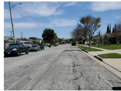
Torry Neighborhood Rehabilitation Project – Before
