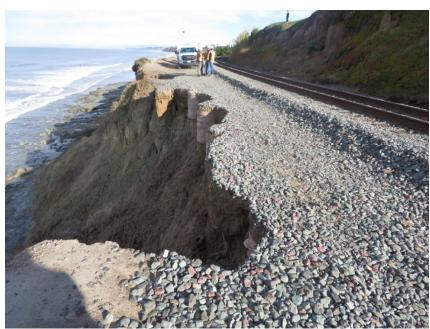
Photo 3: Bluff Slide Thanksgiving 2019 Resulting from Surface Drainage over Bluffs.
