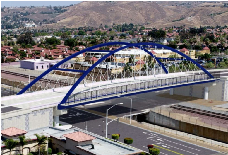
Figure 1 - Steel Tied Arch Network Bridge Overcrossing Looking Southeast
