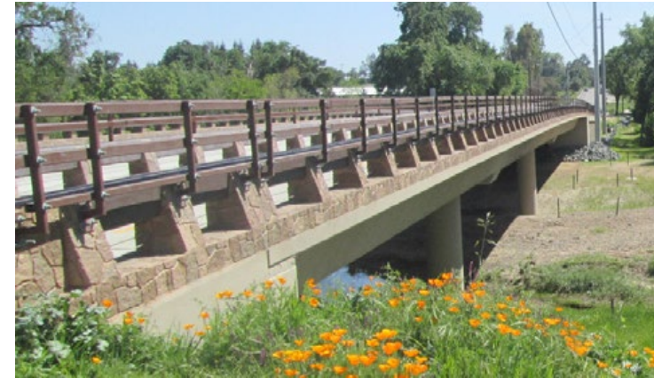
Placer County Cook-Riolo Bridge Replacement
