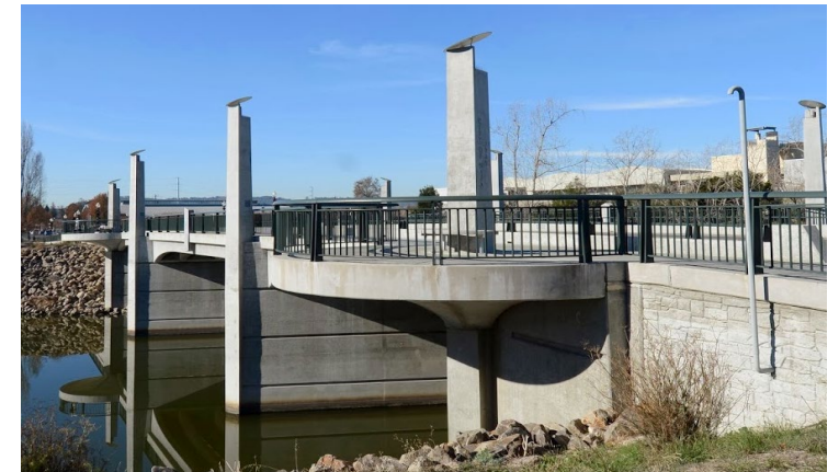
City of Napa First Street Bridge Replacement
