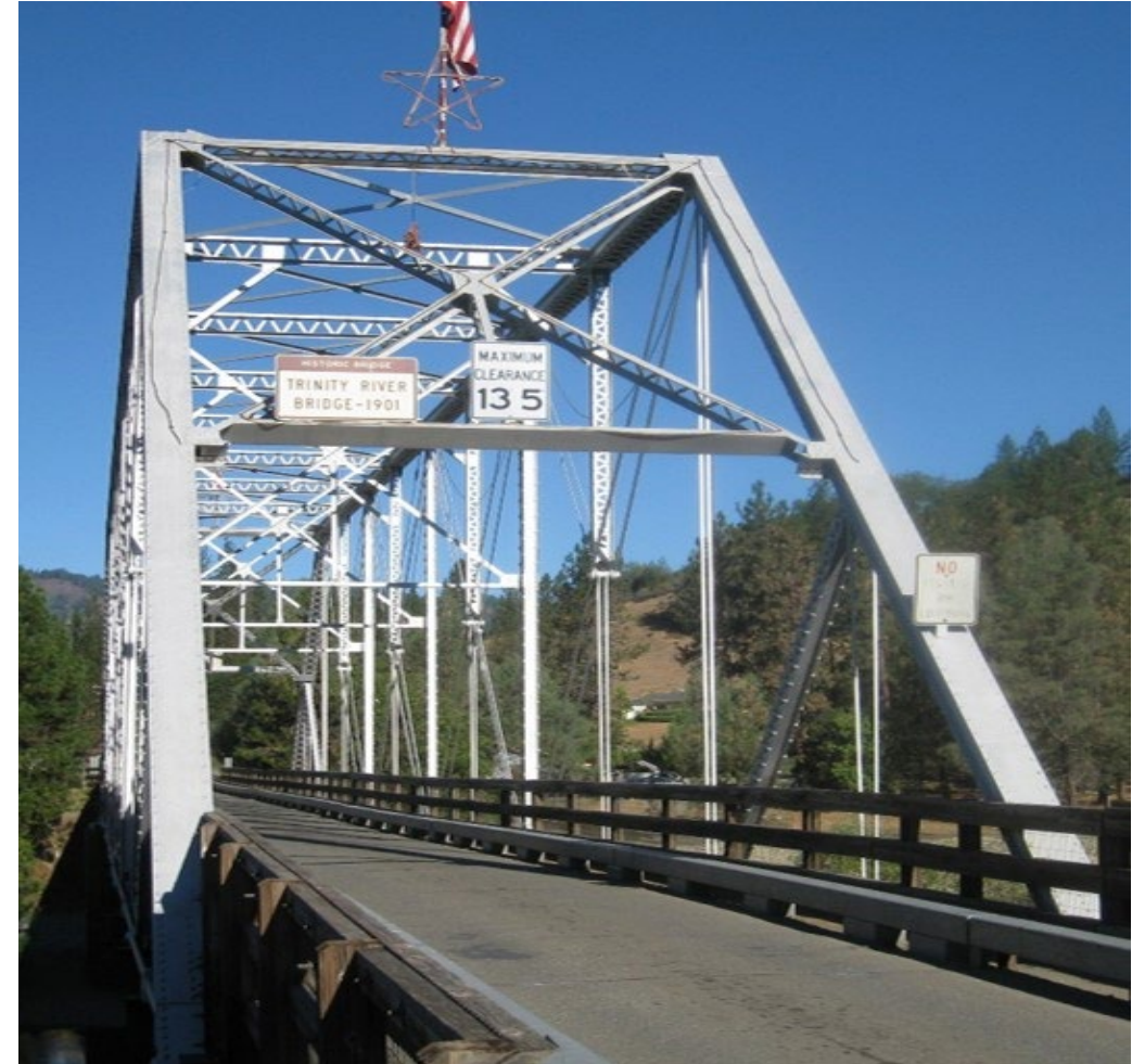
Trinity County Turnpike Road Bridge Painting
