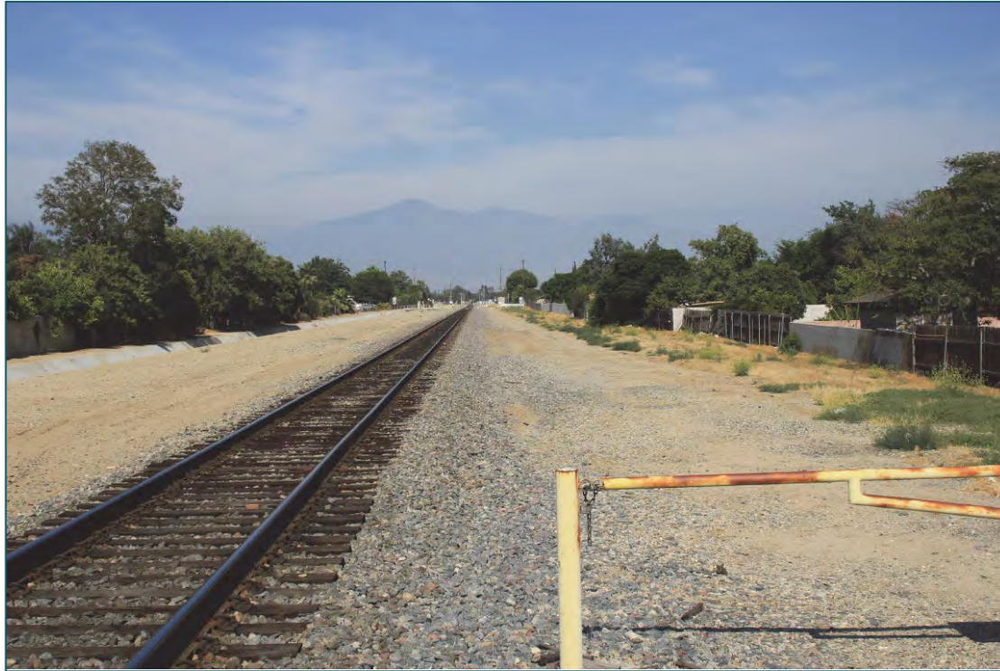
San Bernardino County Metrolink Double Track Project $56.3 million (construction)
