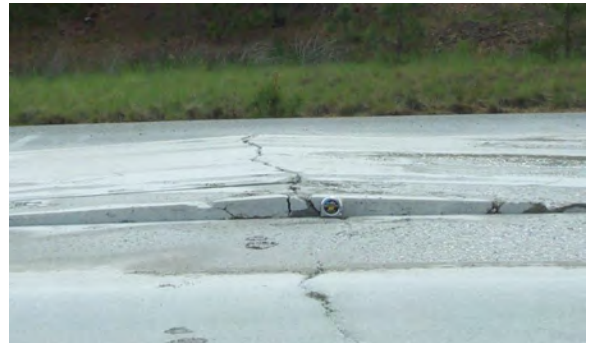
Figure E3. Example of concrete blowup.
