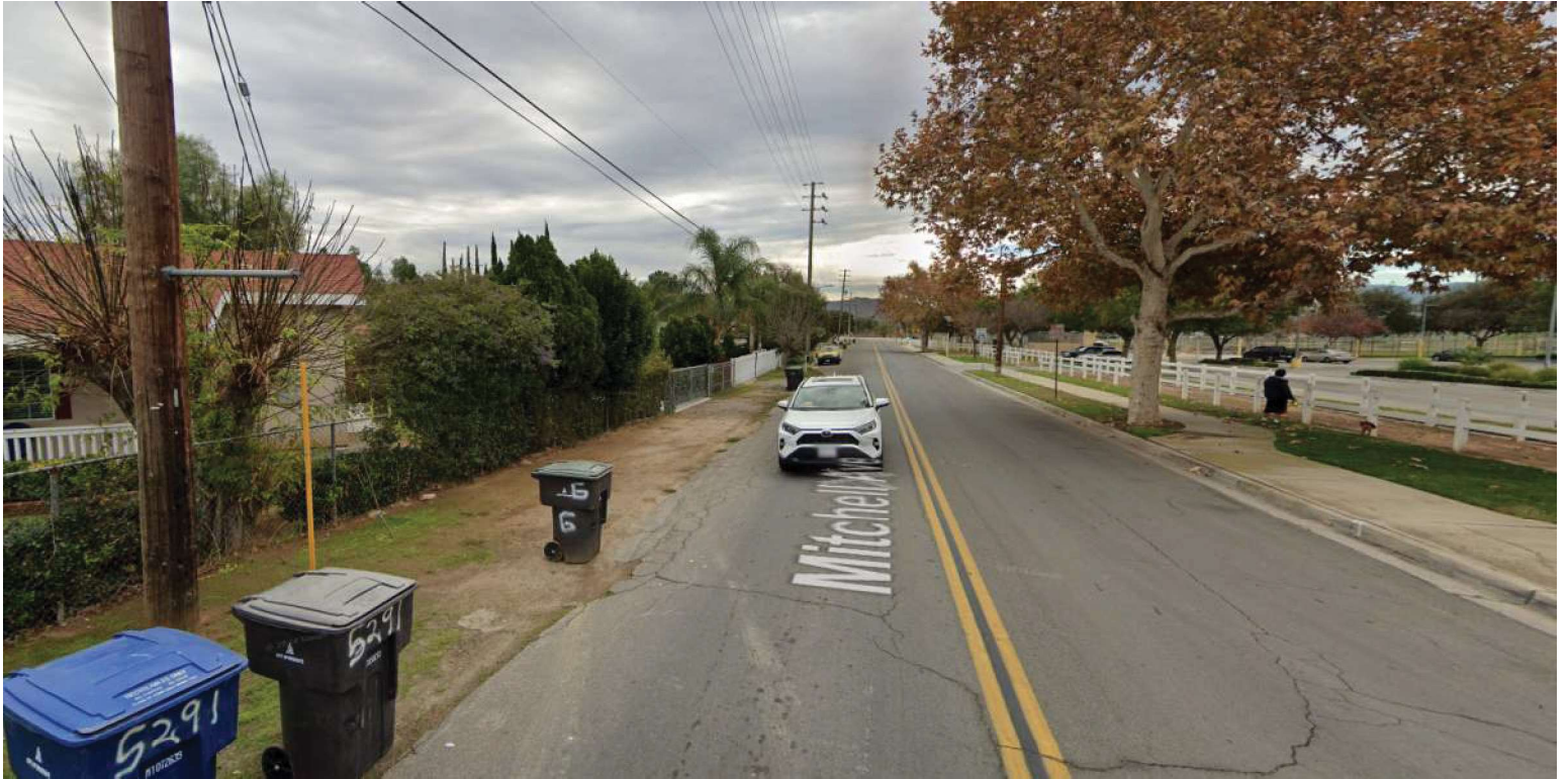
Looking at the south east corner of Mitchell Avenue and Gramercy Place, adjacent to La Sierra Park. This will be the proposed location of a curb ramp and the continuation of the sidepath gap closure towards Bushnell Avenue.
