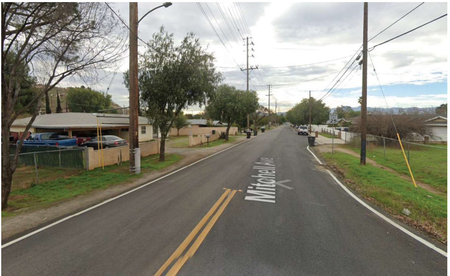
Looking south on Mitchell Avenue from the Campbell Avenue intersection. The first sidepath gap extends 0.37 miles south from Campbell Avenue south to Gramercy Place. Sidewalks are inconsistent, and mostly absent.
