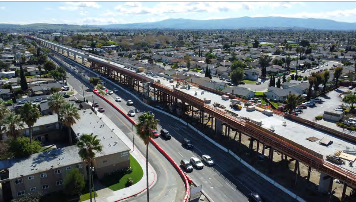
EBRC Light Rail Extension Aerial Guideway Construction
