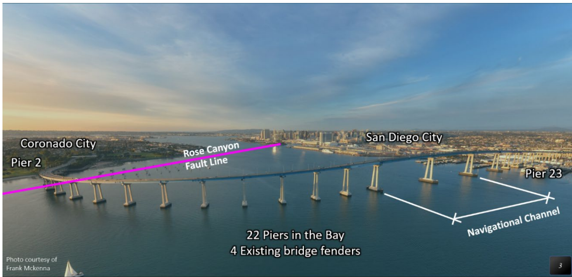
Figure 2: Overview Aerial Photo
