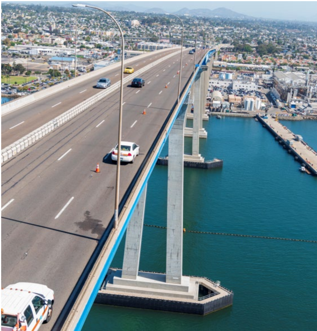
Figure 11: Aerial View of Bridge Lanes
