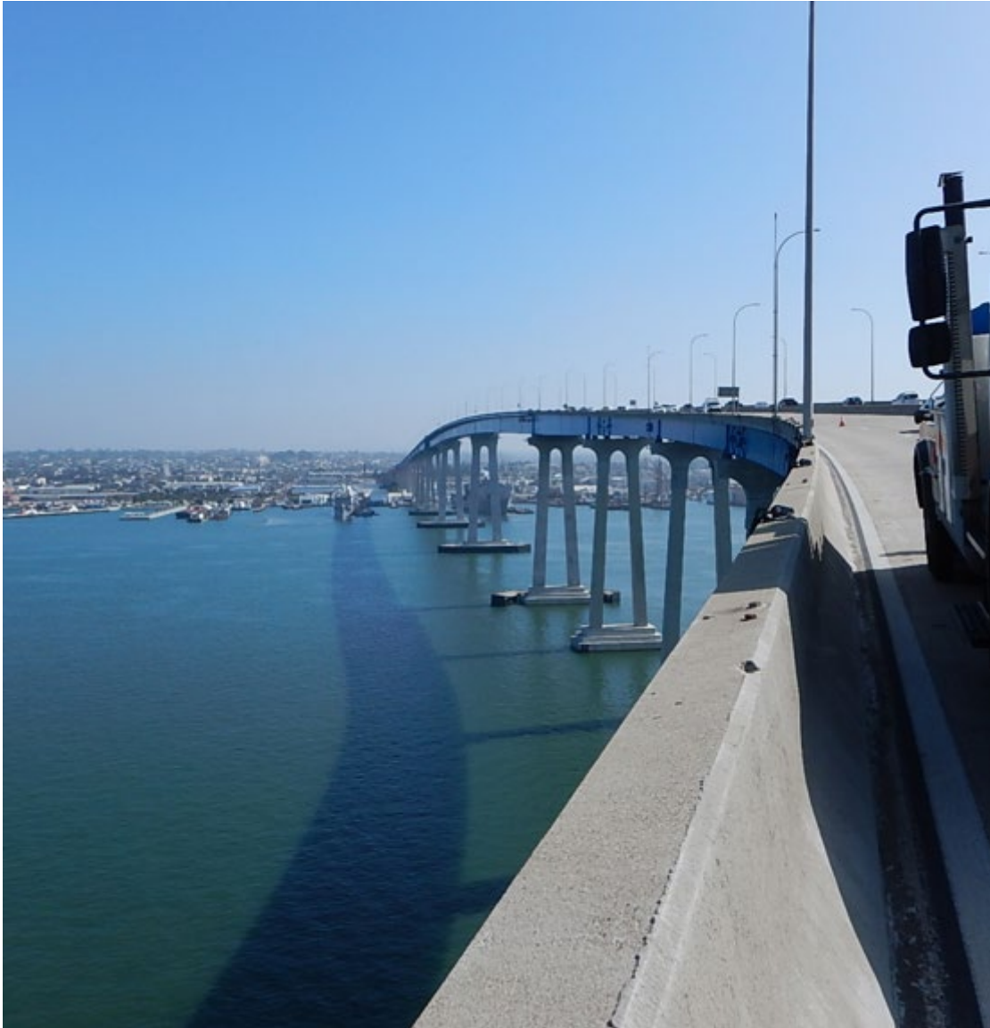
Figure 10: View Along Bridge Rail
