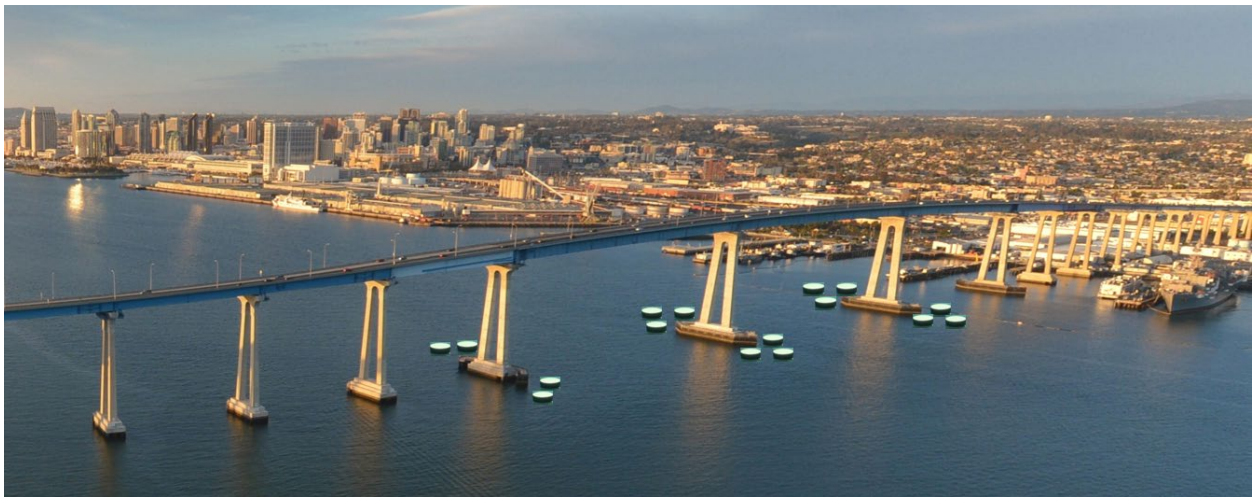
Figure 6: Alt 2– Cofferdam Dolphin Rendering
