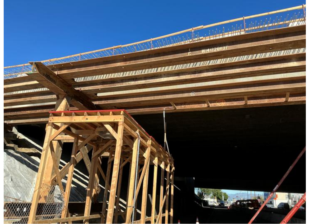
Main St falsework (bridge supports structures) installation
