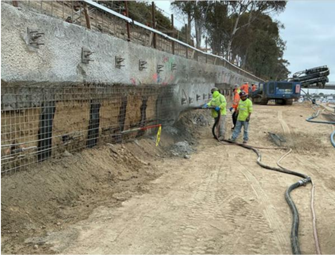
I-105 retaining wall construction
