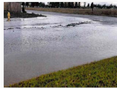
Olivehurst Roadway Project
