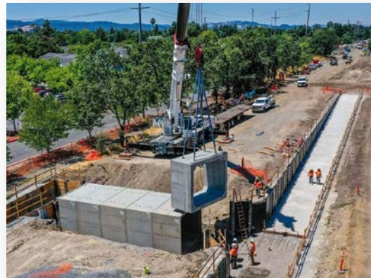
Sonoma-Marín Area Rail Transit (SMART) Windsor Rail Systems Project
