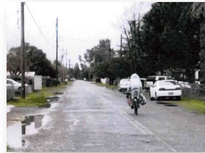
Olivehurst Roadway Project
