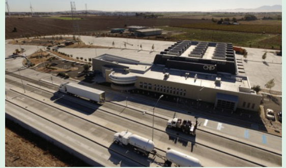
Modern Eastbound Scales, constructed in 2012
