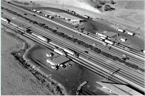
Aging Westbound Scales, constructed in 1958
