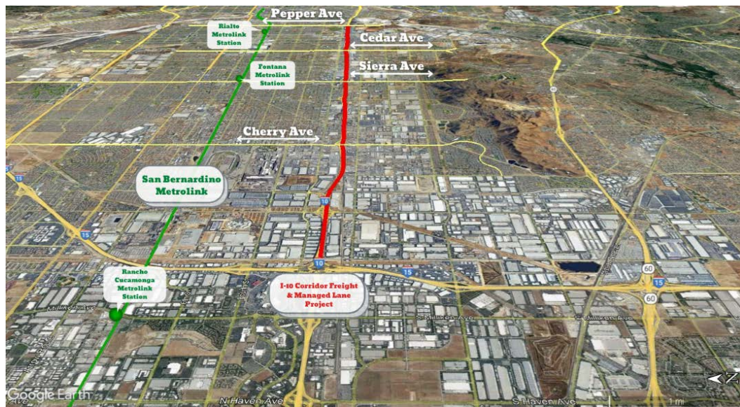
Oblique Aerial of I-10 Segment (in red) looking from west to east across I-15.
