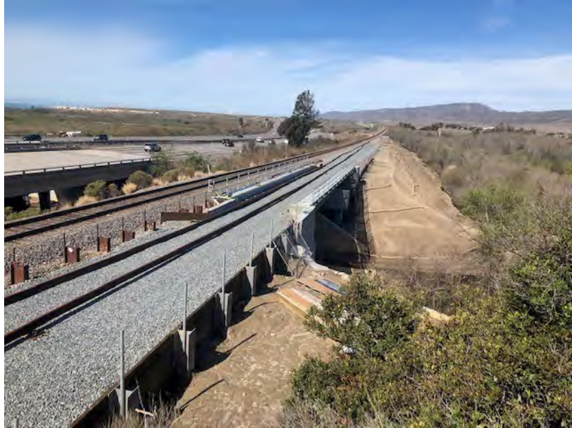
Figure 5: Current construction progress on NAVFAC bridge 218.0 replacement.
