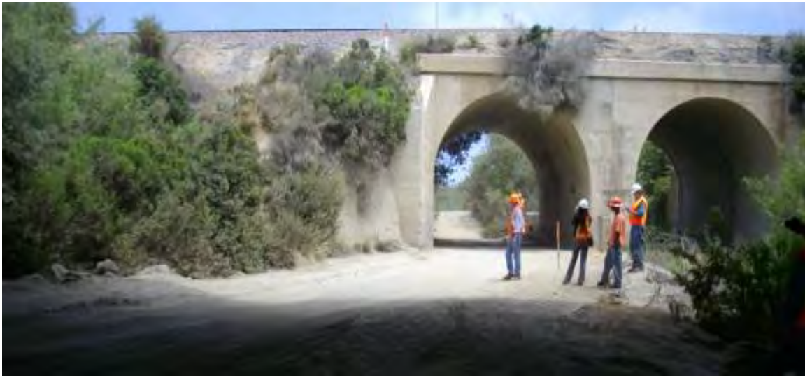
Figure 1: Photo of Existing Br. 218 constructed in 1913 (currently being replaced by NAVFAC)
