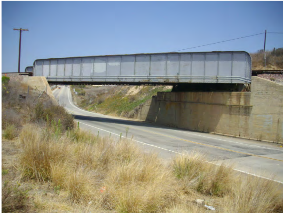
Figure 4: Las Pulgas Road bridge at MP 217.3
