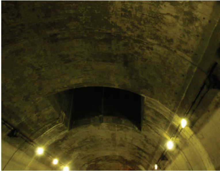
Figure 20: Presidio Tunnel ventilation shaft
