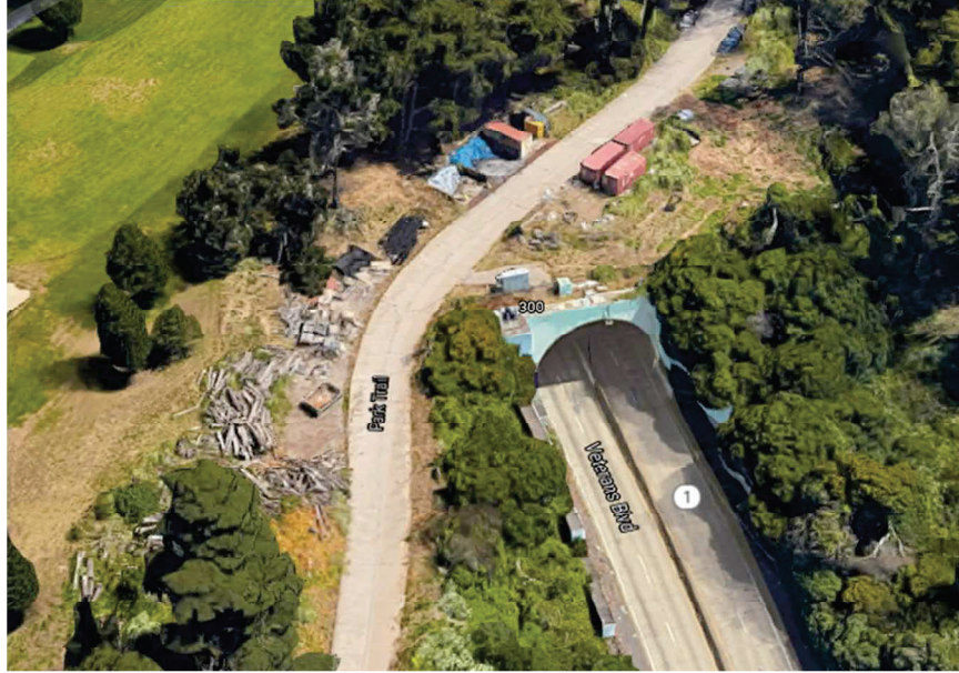
Figure 18: Presidio Tunnel south portal (source: Google Maps)
