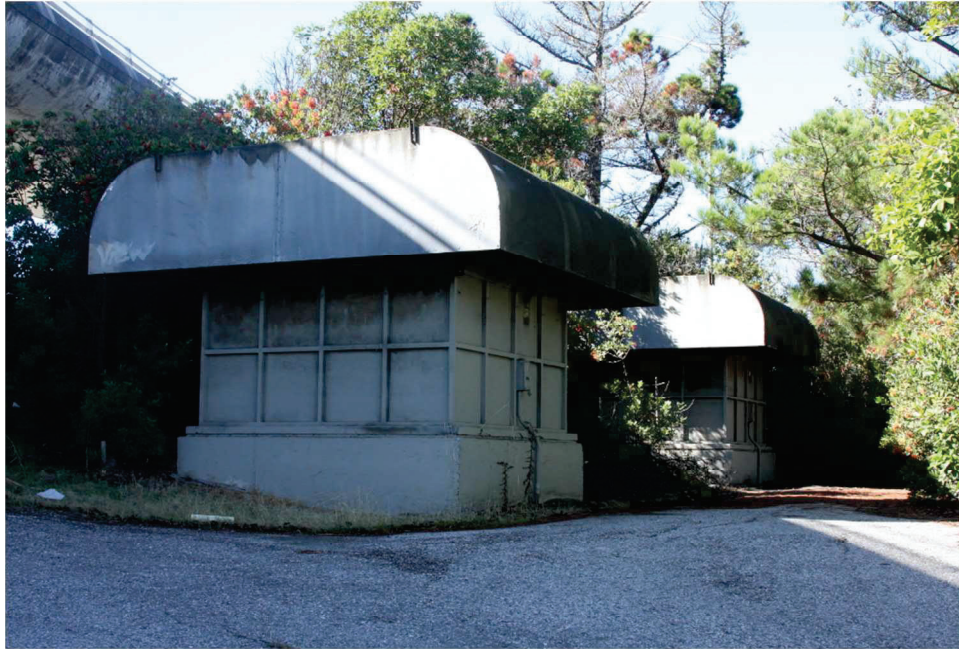
Figure 6: 92-280 Tunnel (South Connector Undercrossing) ventilators
