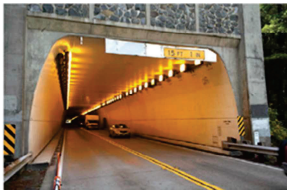
Figure 7: RCT north portal
