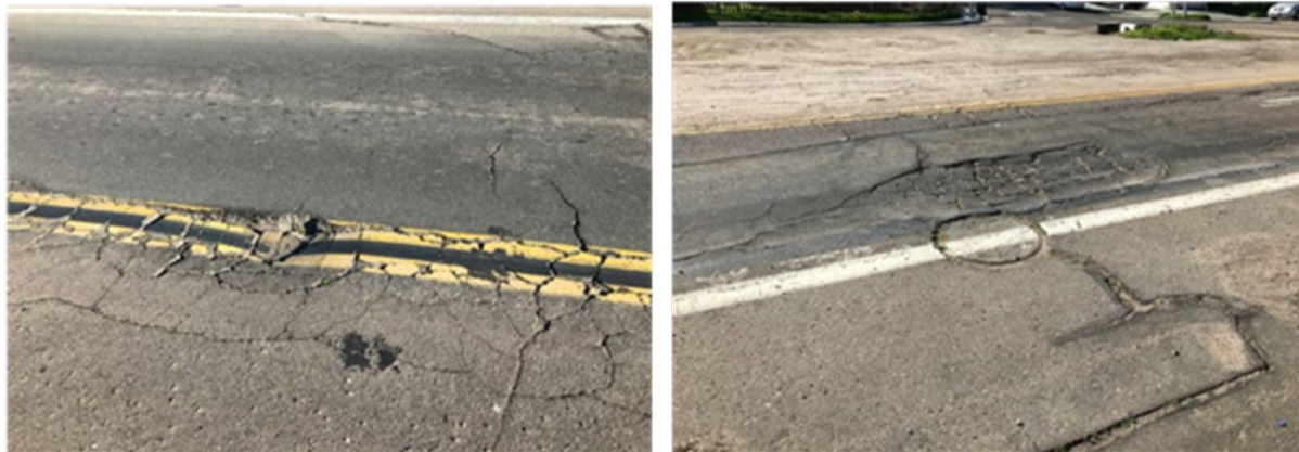
Figure 18: Existing deteriorating pavement on Streamview Drive
