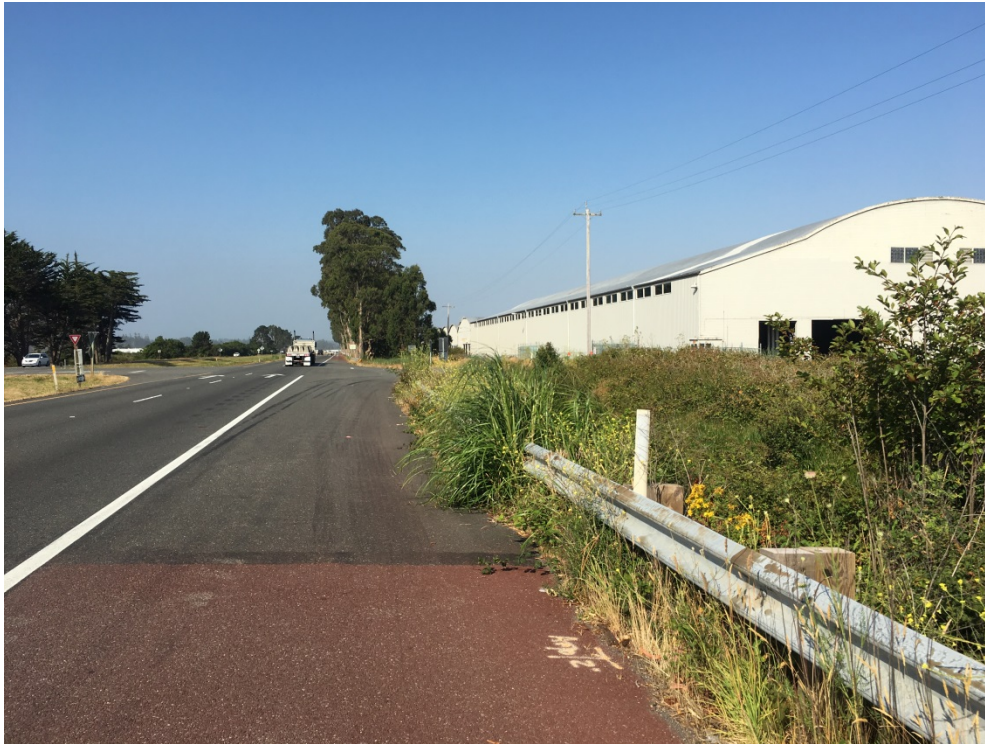
Former lumber mill along the corridor at which Humboldt Bay Trail South will leave the rail corridor and traverse the existing levee west of 101. The red colorized highway shoulder ends at each intersection (and potential conflict point) along the Safety Corridor.
