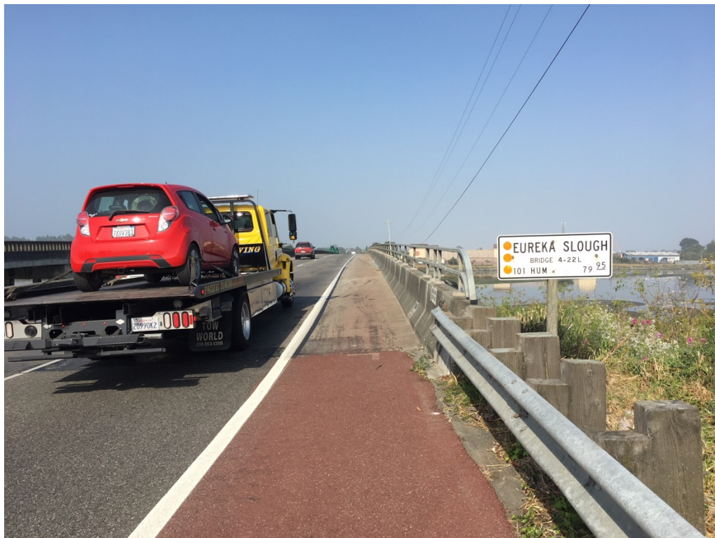
Non-motorized users must currently traverse the narrow Highway 101 Eureka Slough bridges adjacent to fast moving motor vehicles.
