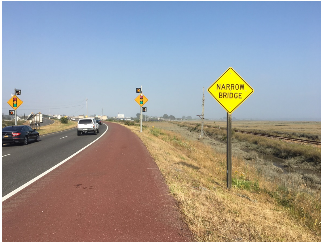
The approach to the Highway 101 bridges over Eureka Slough with the rail corridor just west.
