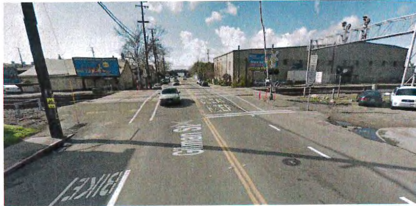
Gilman Street at UPRR Tracks, looking west
