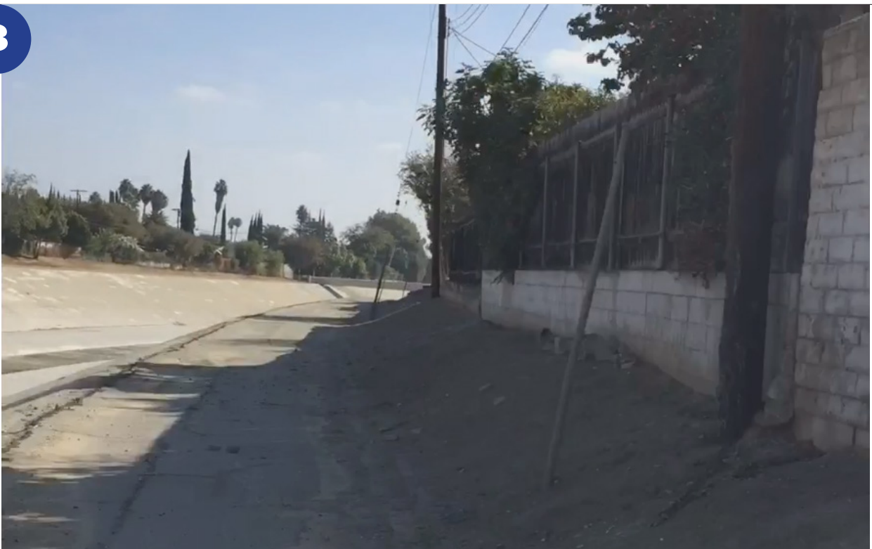
Unimproved Project Area - Along proposed Greenway ROW - Constrained width section between Wilbur Ave and Yolanda Ave. Note poor quality of maintenance road without official public access; lack of railings; and encroaching dirt and utilities.
