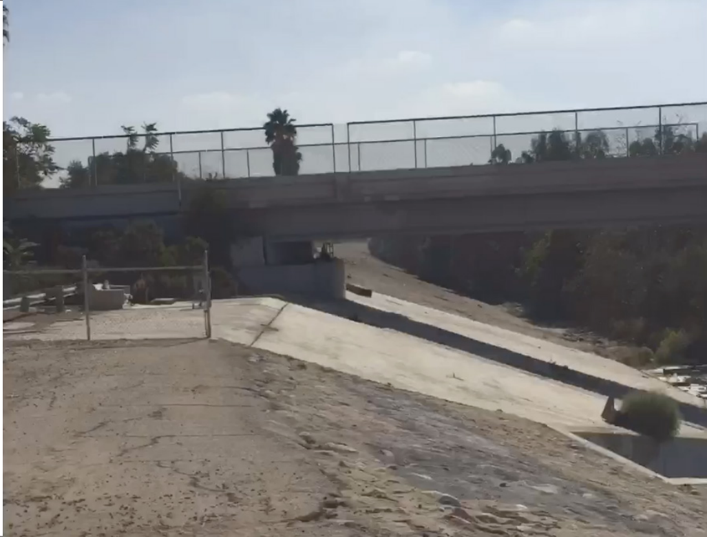
Unimproved Project Area - At Metro Orange Line Busway bridge - Looking east. Note lack of level path of travel requiring undercrossing.
