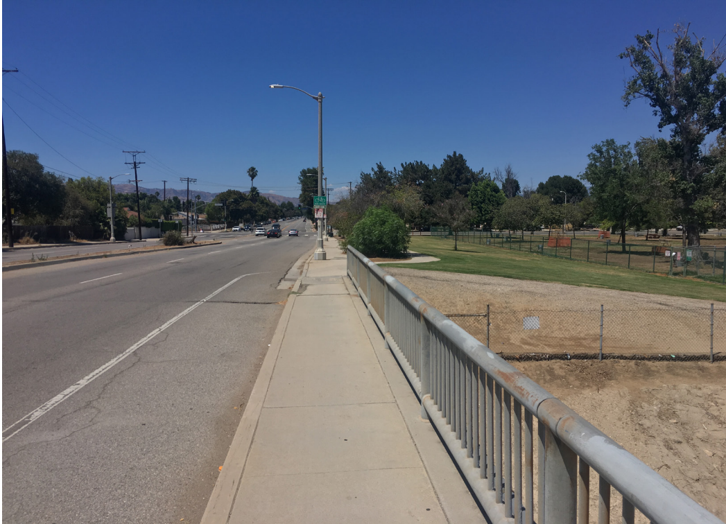
White Oak Ave bridge looking north. Project proposes a two-way Class IV protected cycletrack on this (east) side to transfer LA River Greenway from the south bank to the north bank. Note the end of the bridge where a raised-table mixing zone is proposed for the junction of the sidewalk and the LA River Greenway and the N-S bike path that is proposed to be expanded to a two-way path.
