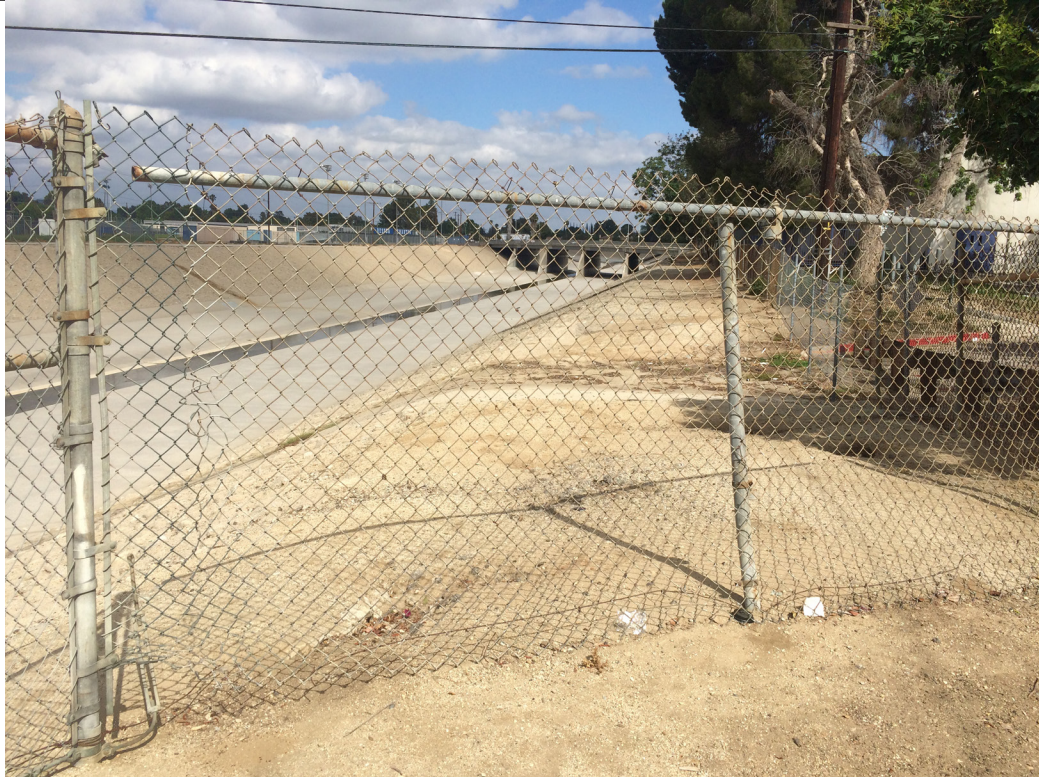
Unimproved Project Area - Etiwanda Ave/Reseda Park, at bridge - Looking east. Note chain link fence and unimproved dirt ROW without official public access or improvement.
