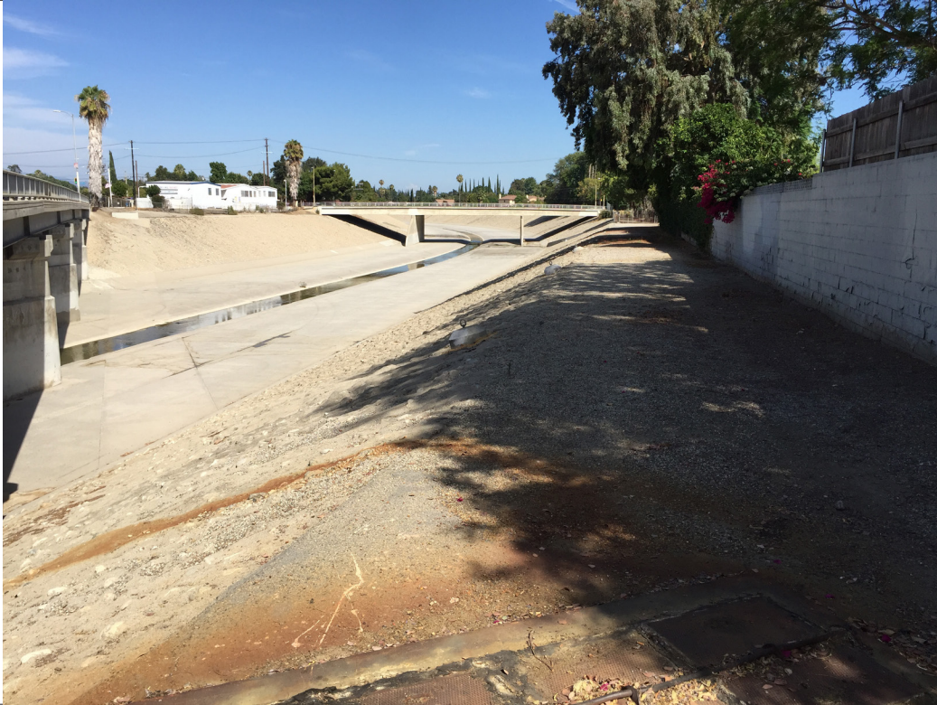
Unimproved Project Area: In LA River Flood Channel at Victory Blvd looking southeast towards Lindley Ave.
