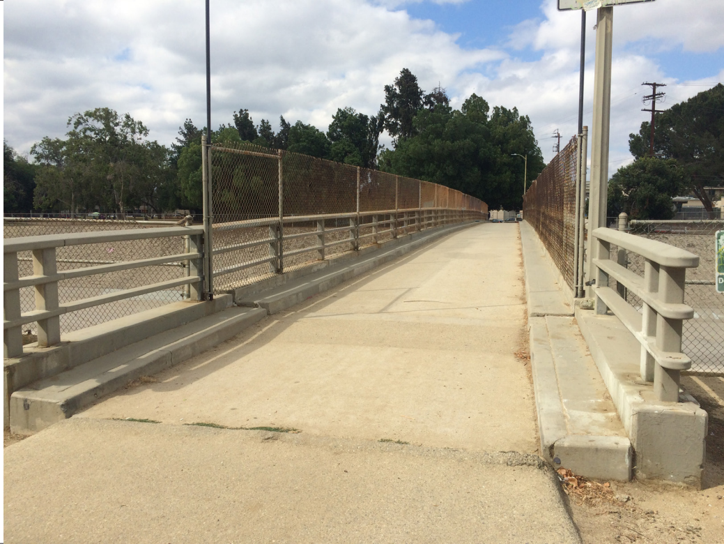
Existing Pedestrian Bridge - Etiwanda Ave/Reseda Park Pedestrian Bridge - Looking north. Project will add conflict markings and signage.
