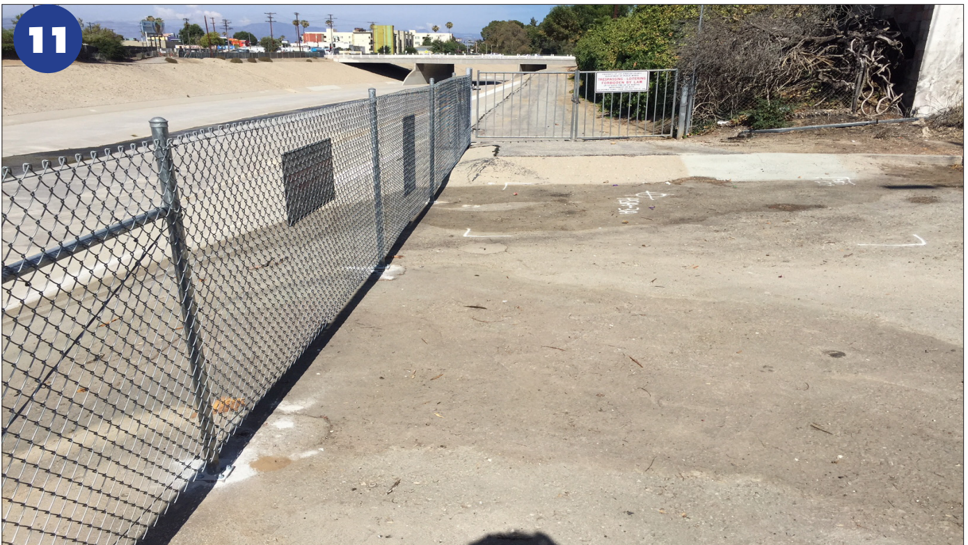
Amigo Street end, south bank of LA River looking east. Note fencing and drainage.
