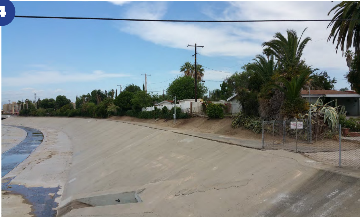
Unimproved Project Area - At Vanalden Ave - Looking east. Note chain link fence, maintenance road without official public access and lacking railing on LA River side.
