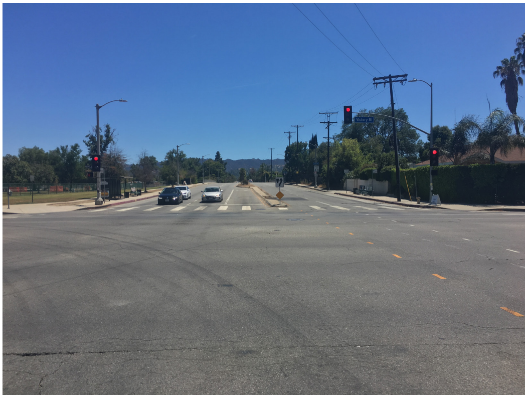
Intersection of White Oak Ave and Victory Blvd looking south. Note lack of bike lanes on northbound approach. Project proposes new Class II bikelanes northbound and a Class IV cycletrack southbound leading to the bridge and continuous Class IV south to Oxnard St.
