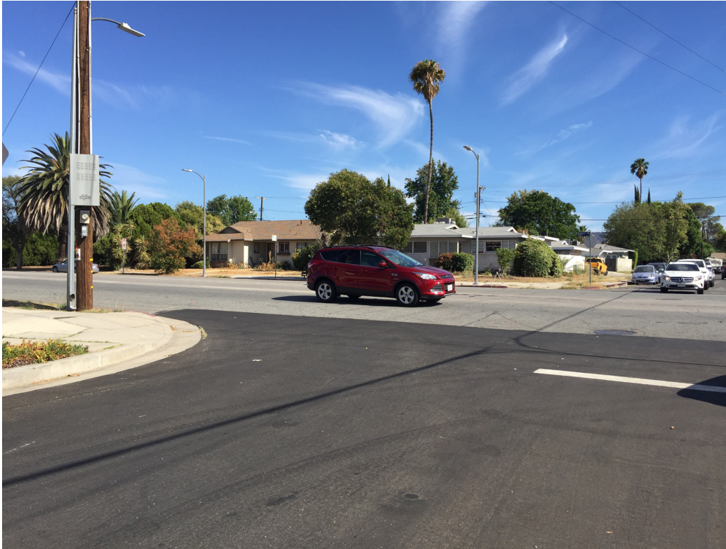
Vanalden Ave/Victory Blvd intersection looking south across Victory Blvd. Note the lack of control for Victory Blvd. The Project would place a new full signal at this intersections, enabling safer crossings of a street with a 45 mph posted speed limit.
