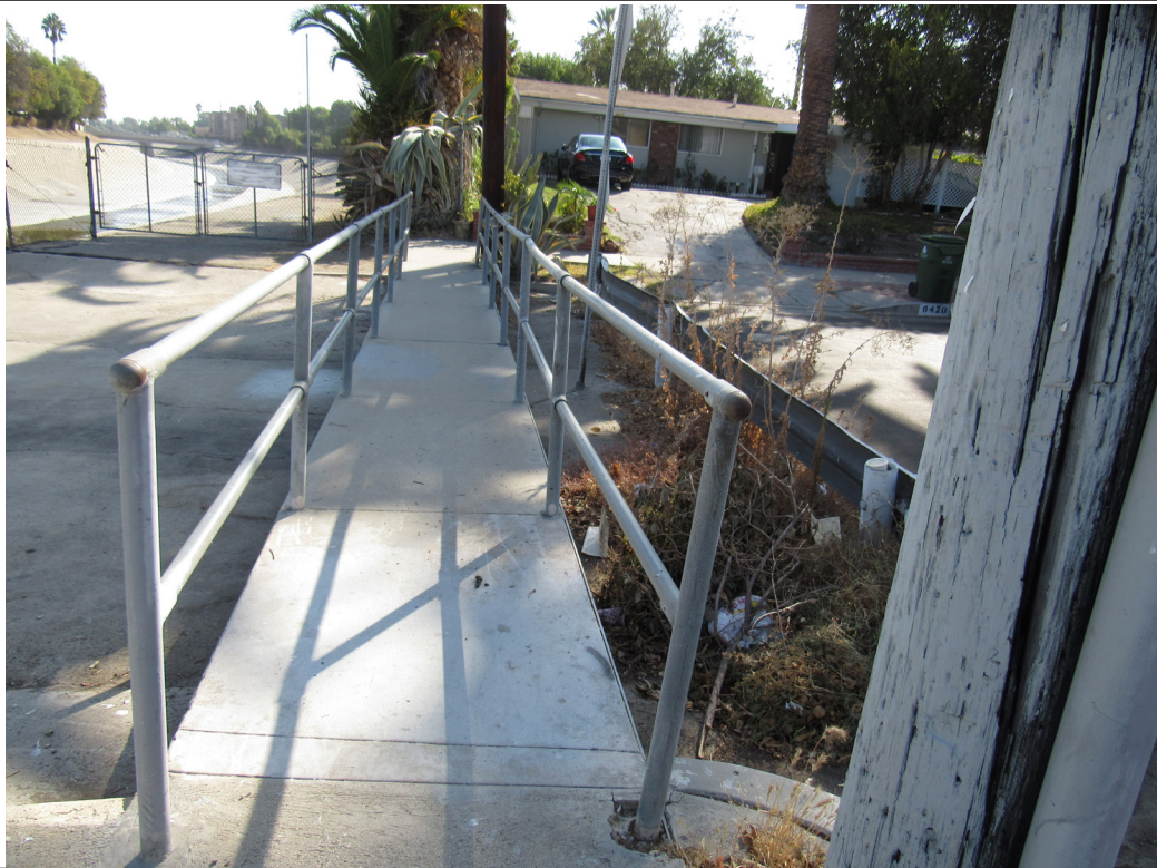
Unimproved Project Area - Existing stormwater management culvert at Vanalden Ave - Looking west. Project will redesign street end by completely capping the section with the proposed greenway and adding ADA access ramps.
