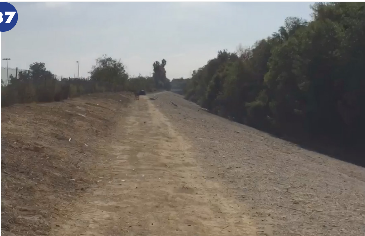
Unimproved Project Area - Proposed Greenway ROW through Sepulveda Basin btwn Orange Line & Balboa Blvd - Looking east. Note dirt maintenance road without official public access.
