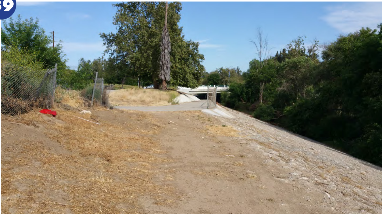
Unimproved Project Area - Just west of Existing Bikeway at Balboa Blvd - Looking east. Note dirt maintenance path and ripped-open chain link fence allowing unofficial access to flood channel.
