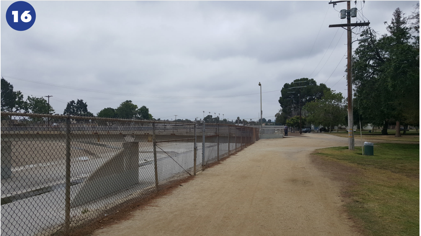
Unimproved Project Area - Reseda Park - Looking west at Greenway path which will run down current maintenance path adjacent to fence. Note chain link fence and a lack of official public access to channel.
