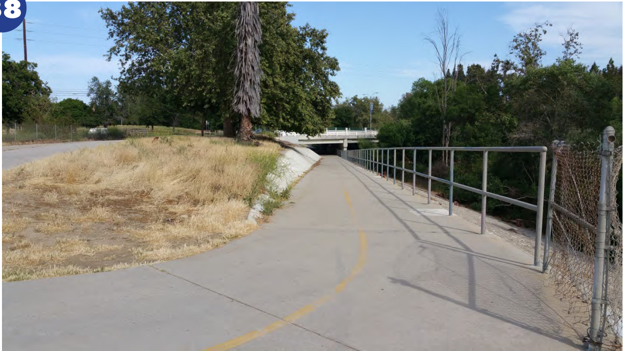
Existing Bikeway Underpass - At Balboa Blvd - Looking east
