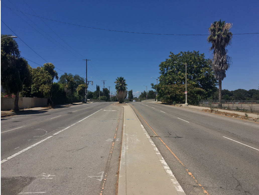
White Oak Ave south of bridge looking north with recreation area on the right. The concrete island will be removed and new Class IV protected cycletracks will be implemented.
