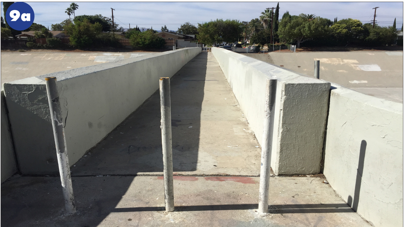
Amigo Pedestrian Bridge. Note bollards blocking cycling access.
