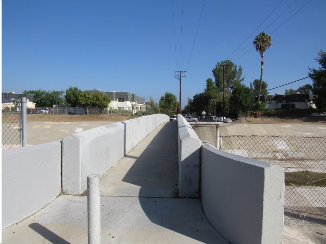
Unimproved Project Area - Existing Vanalden Ave Pedestrian Bridge (note bollard) - Looking north. Project will remove bollards and add conflict marking paint and signage.
