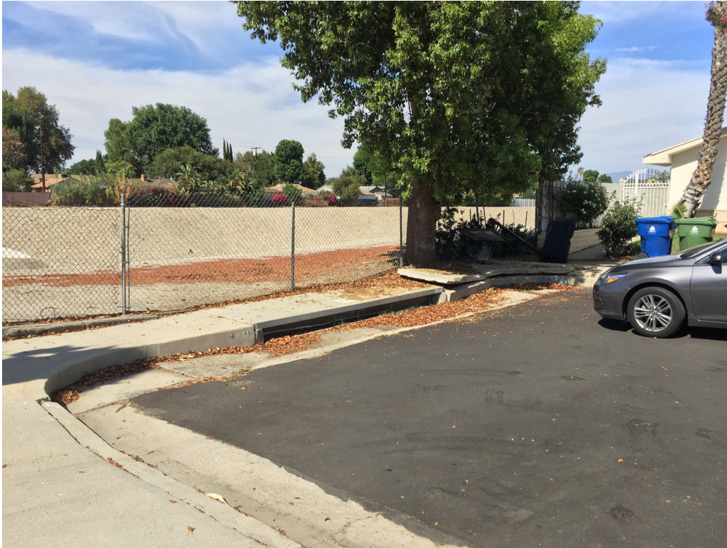
Zelzah Street End, south bank of LA River. Proposed access point for LA River Greenway. Note lack of ADA access.
