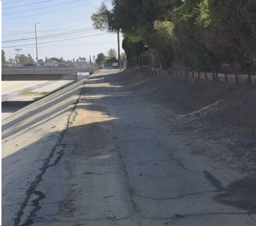
Unimproved Project Area - Along proposed Greenway ROW just west of Wilbur Ave - Looking east. Note unimproved maintenance road without official public access; encroaching dirt; and lack of protective railing.
