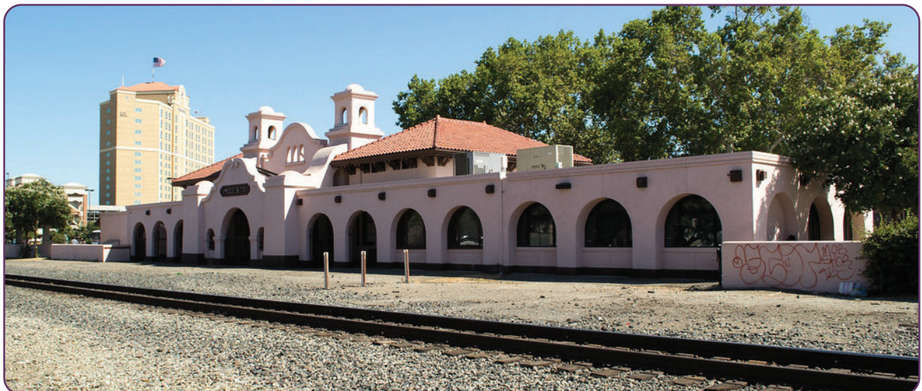
Photo of existing Modesto Transit Center
