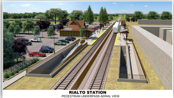
Figure 1 (above) – Proposed Double Track, New South-Side Platform, and Pedestrian Underpass at Rialto Station
