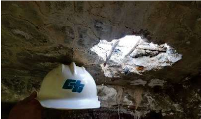
Through Deck Hole at Abutment 8 Span 7
