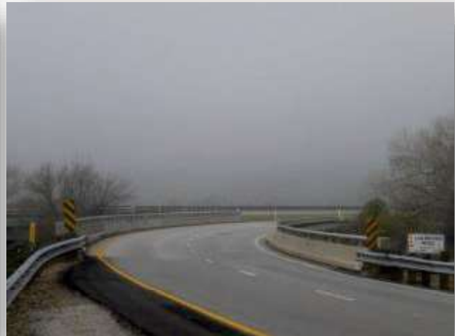
Looking west toward Abutment 1
