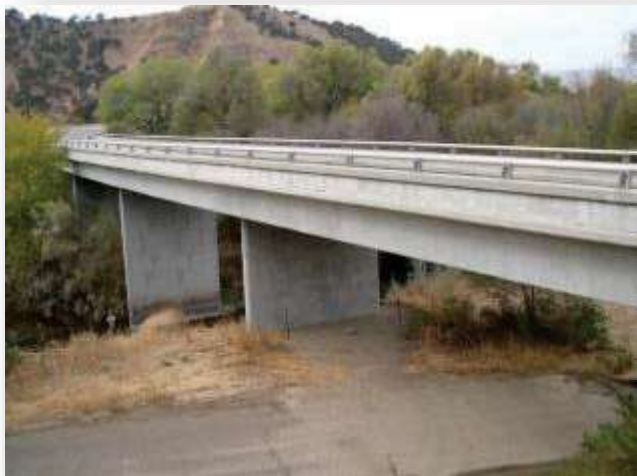
Looking northwest toward the left edge of bridge
