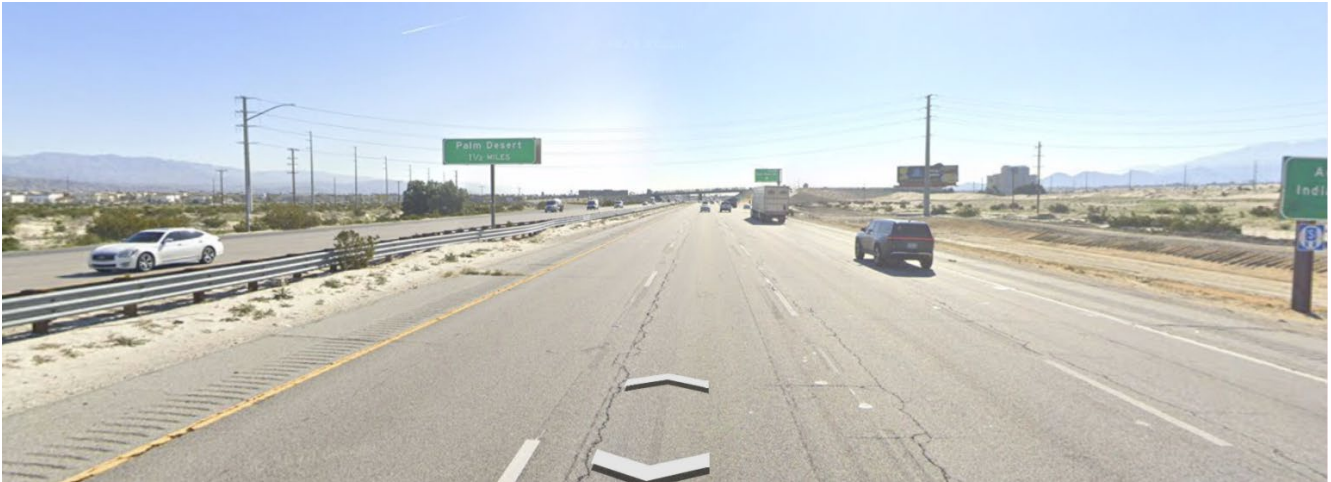
Figure 17. Alt. 6.0—baseline concept: sample image of roadway conditions (not representative of entire roadway)
