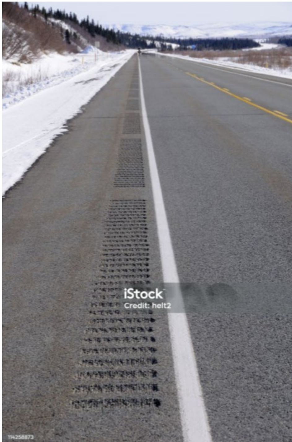
Figure 19. Other Design Consideration (M-01)—baseline concept: traditional rumble strips
