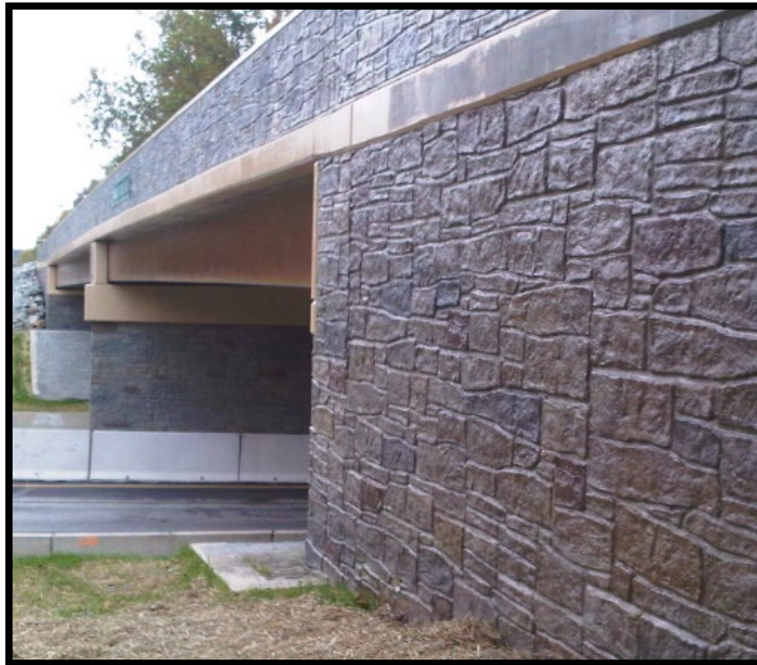
Example of texturized and stained overpass
