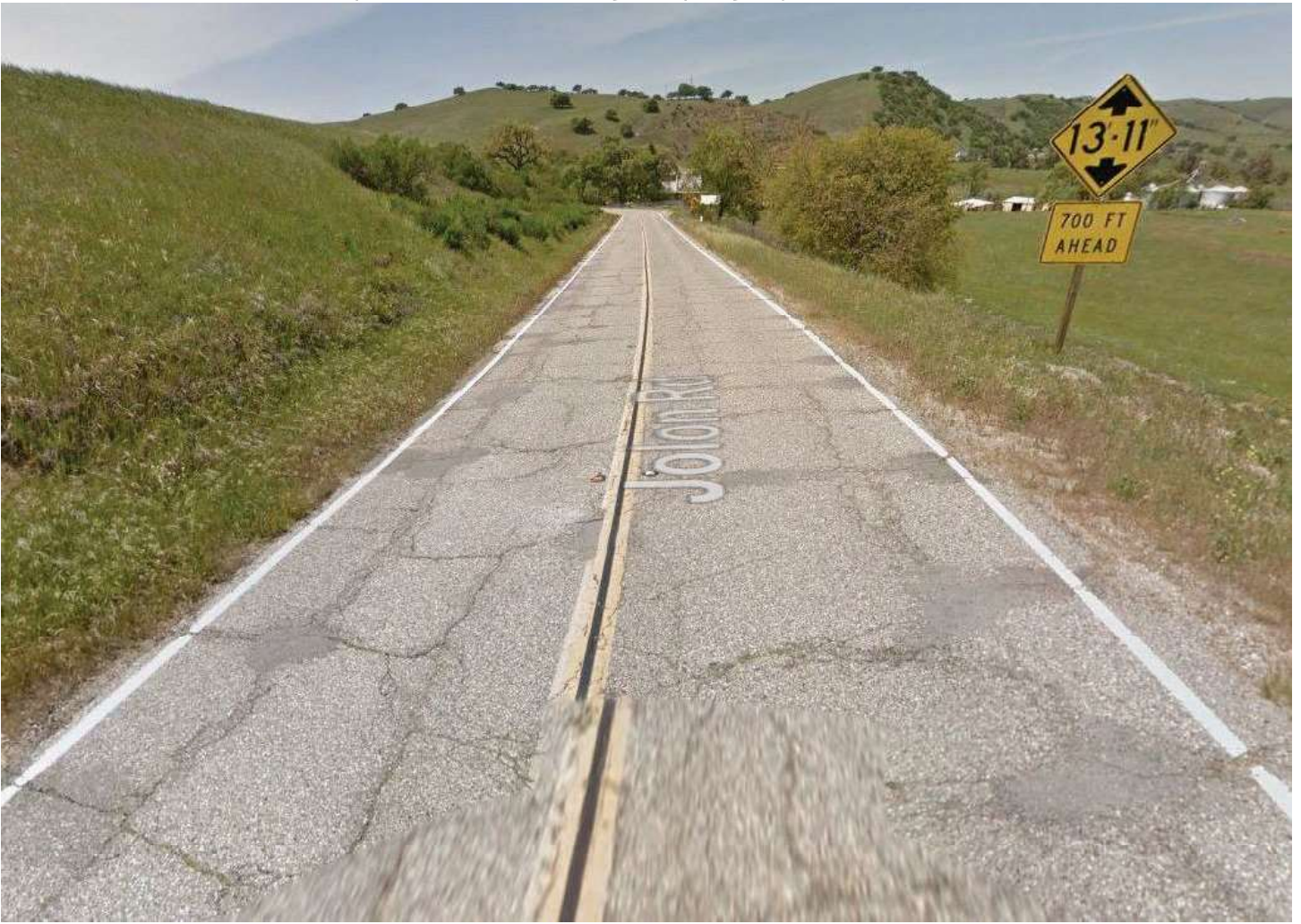
Figure 1: Northbound off-ramp where potential for complete streets improvements exist
