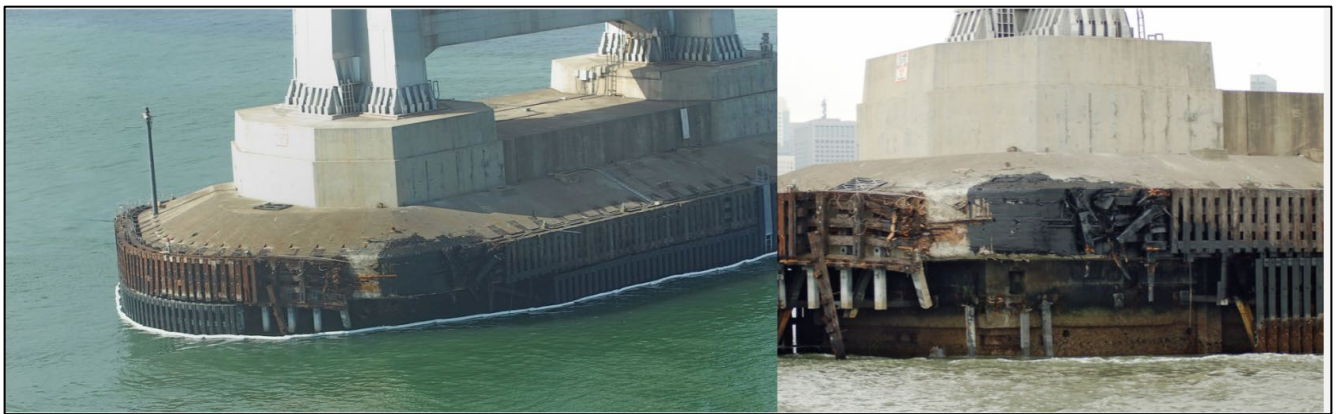
Photos of the damage to SFOBB Pier W5 after the Cosco Busan allision, 2007
