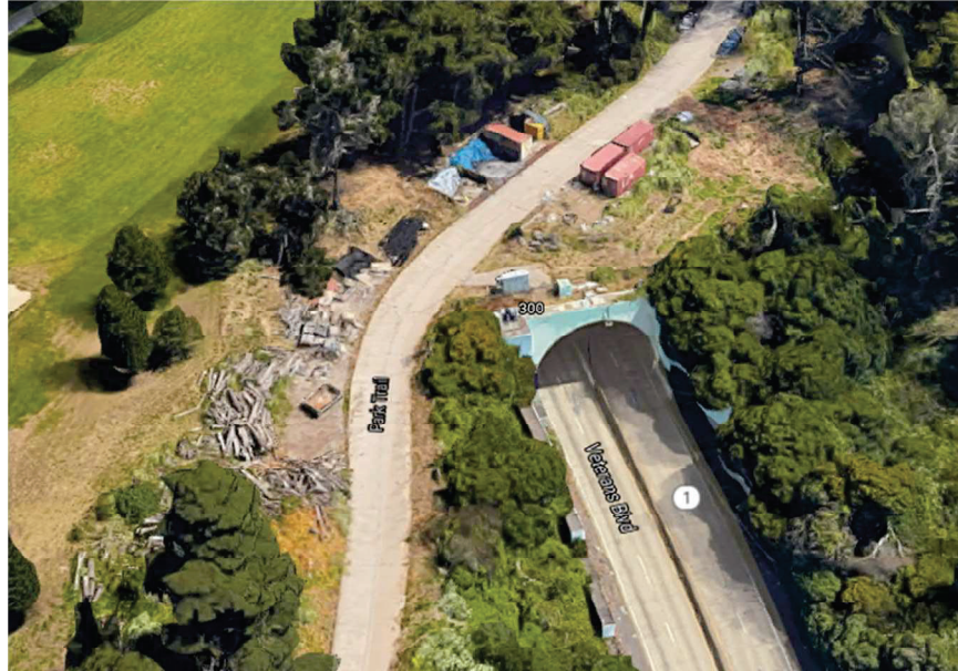
Figure 18: Presidio Tunnel south portal (source: Google Maps)
