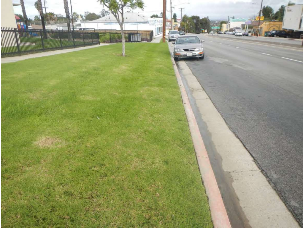
Figure 3 Site 3, Biofiltration Swale, North View
