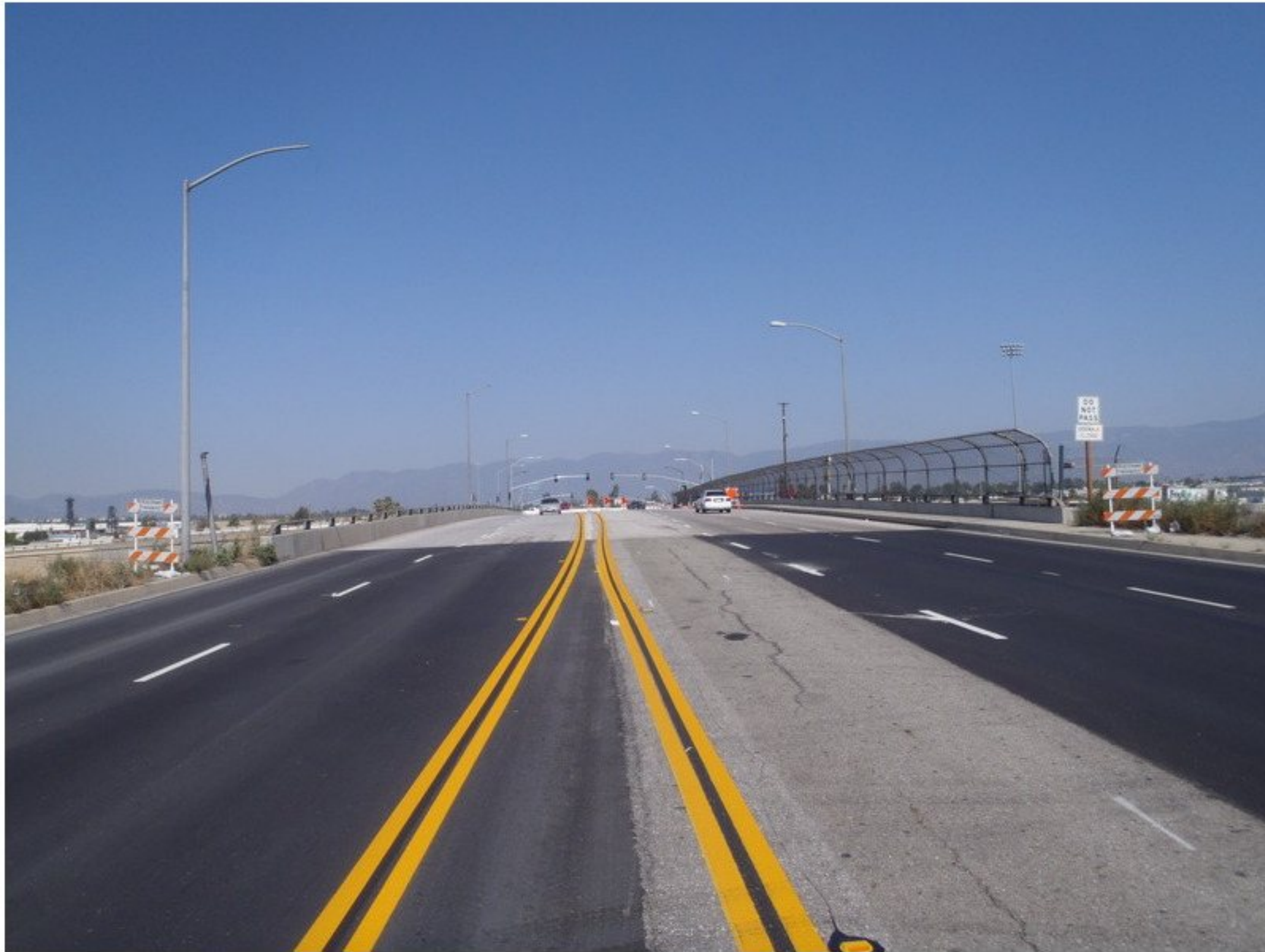
Photo No. 1 Routine deck view looking north on Riverside.
