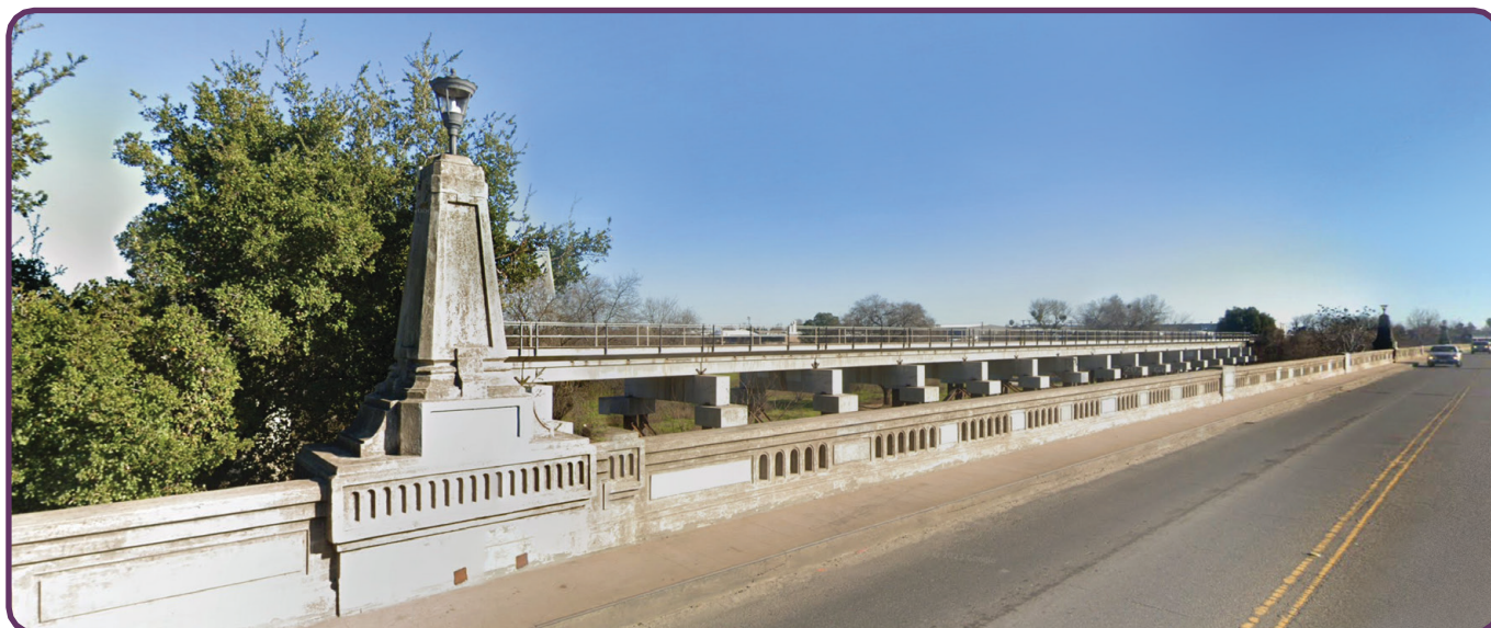
Existing UPRR Tuolumne River Bridge as seen from Seventh Street
